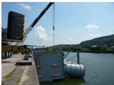
Energie Fleuves installs the first water turbines on the River Meuse
